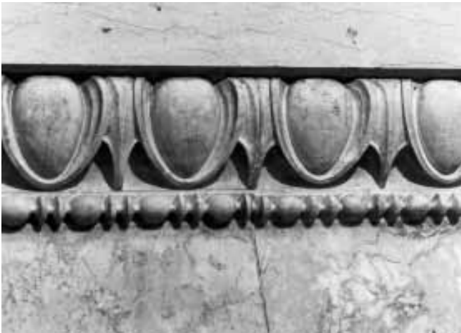
Detail of marble. The marble for the building was cut and carved in Buffalo, New York, in the shops of Lautz Company, the marble contractor. As with the granite, the Society's representatives had to inspect the work rigorously to ensure its quality.
