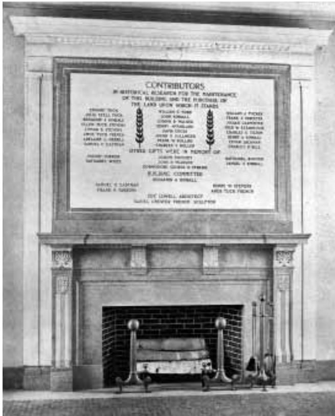
Contributors' tablet. Problems involving the production of the marble tablet over the reading room fireplace, with its inlaid bronze lettering, were among the last of many faced by the building committee as dedication day drew near. New Hampshire Historical Society.
