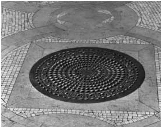
Rotunda floor tiles. Lowell specified marble tiles in the rotunda, Grueby art tiles in the library, and brick-like Mercer tiles in the second-floor gallery. A large number of tiles needed to be reset due to shoddy workmanship detected by Kimball and Sullivan.
