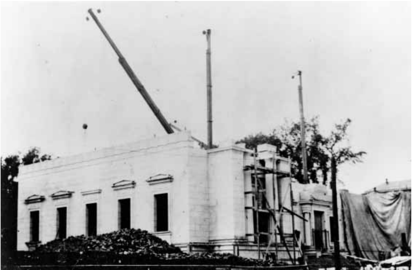
Work on hold for the winter, 1909–10. Progress during the fall was slow, and, despite warnings from Lowell, the roof was not capped before cold weather arrived. In the spring the tarpaulins were thrown aside, and the walls again began to rise toward the cornice. Rough blocks of granite appear over the doorway where the sculptural group is today. New Hampshire Historical Society.
