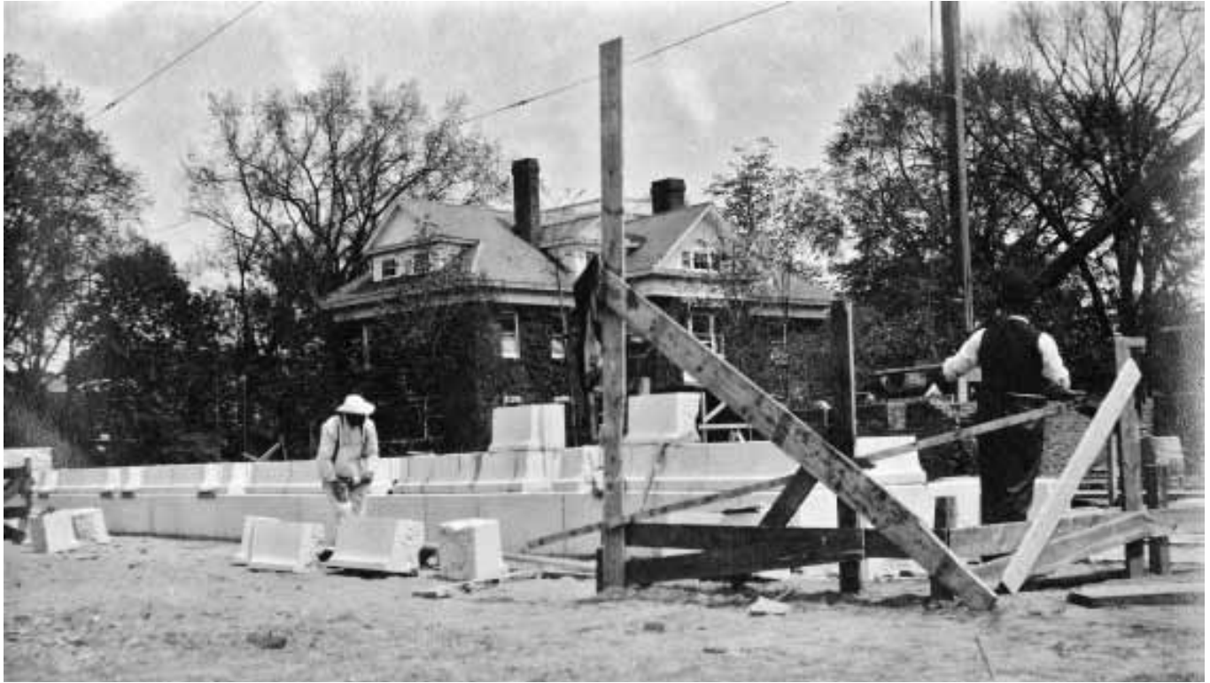
Work underway on the foundation, spring 1909. During the cornerstone laying ceremony, Kimball expressed the hope that “this building of granite, marble, steel and bronze [may] exist forever,” yet a series of problems seemed to threaten its completion. New Hampshire Historical Society.
