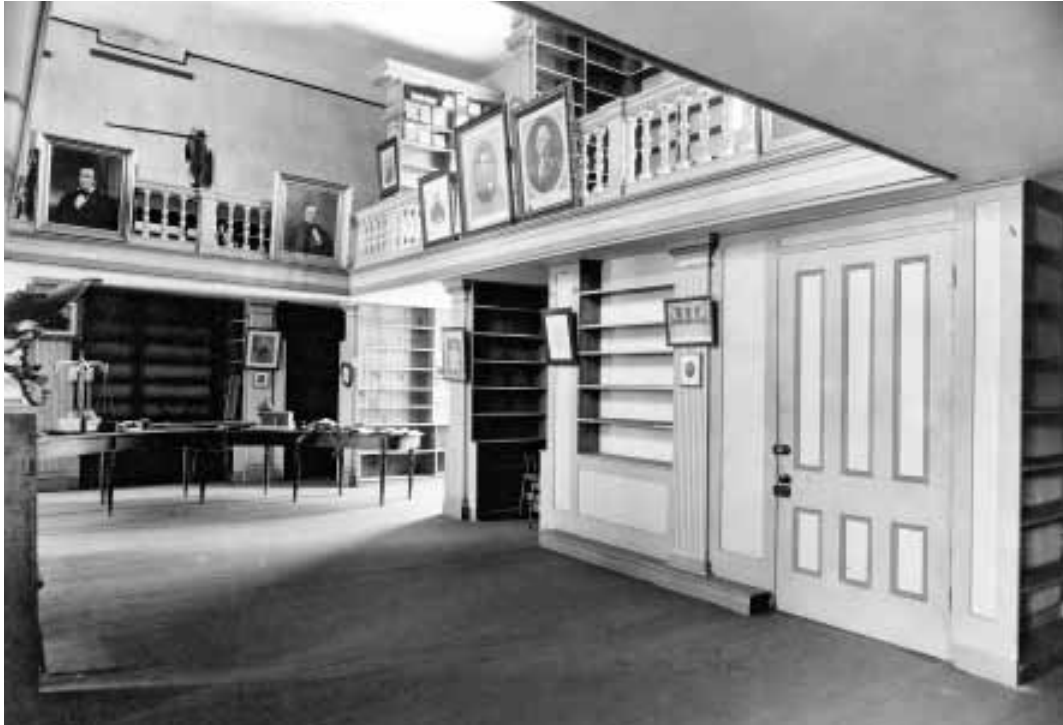
Interior at North Main Street, photographed after the removal of the book collection to the new library, c. 1912. The walls of this building were brick, but its interior was combustible. Although a fireproof vault had been built about 1895, plans were developing by 1900 for a large fireproof addition at this site. New Hampshire Historical Society.
