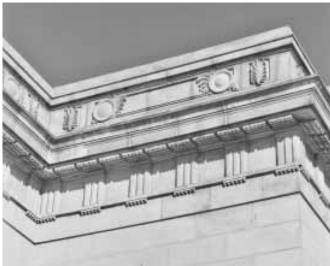
Detail of the Doric cornice with its fragile guttae. "Under Mr. Sullivan's careful supervision, . . . no detail was too trifling to be overlooked, and his painstaking inspection, while necessitating slow progress, made the work when completed a model of excellence" (Concord Daily Patriot, November 23, 1911).
